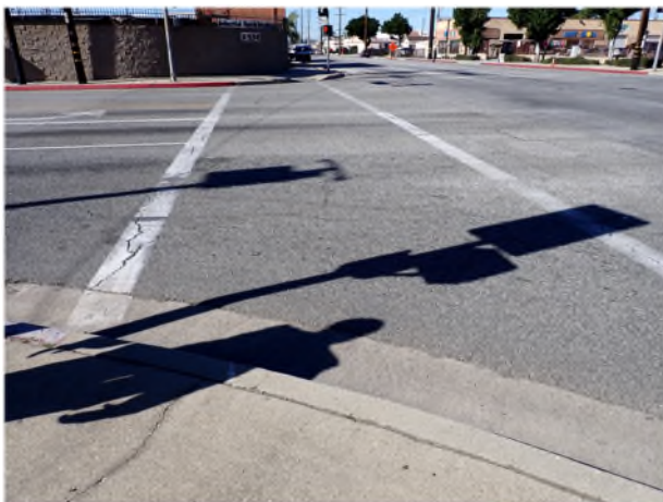
PHOTO NO. 3 – SITE NO. 6 (RUSH ST & MERCED AVE)
