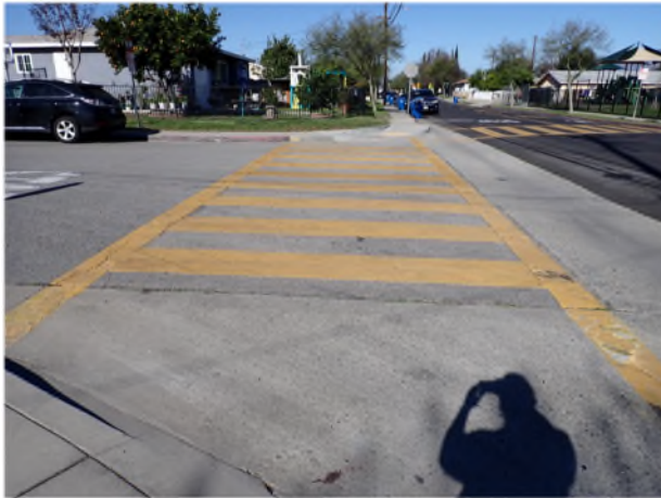
PHOTO NO. 1 – SITE NO. 20 (THIENES AVE & LEAFDALE AVE)
