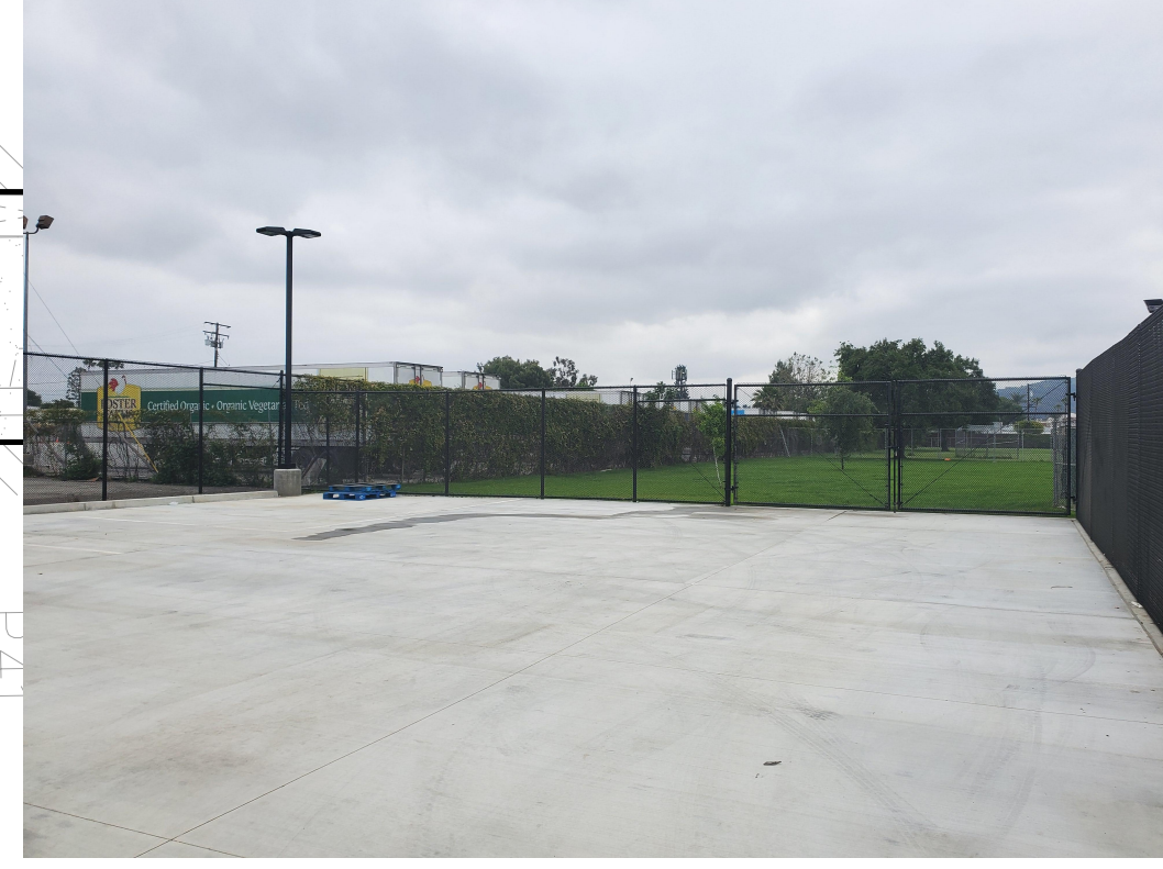
Property perimeter fencing and light standards are provided.
