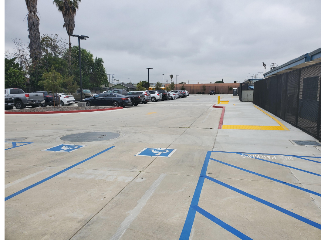
Overview of the parking lot. Note concrete paving, perimeter fencing and light standards.
