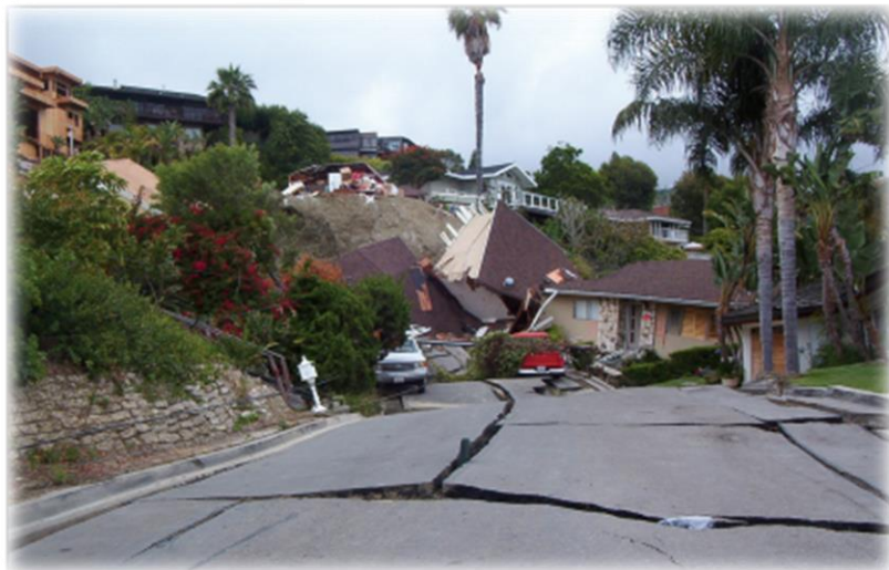
Caption: Bluebird Canyon landslide, June 1, 2005, near Laguna Beach, California that caused 350 homes to be evacuated, of which 15 were damaged or destroyed. The movement was most likely caused by heavy rains in January and February 2005.
