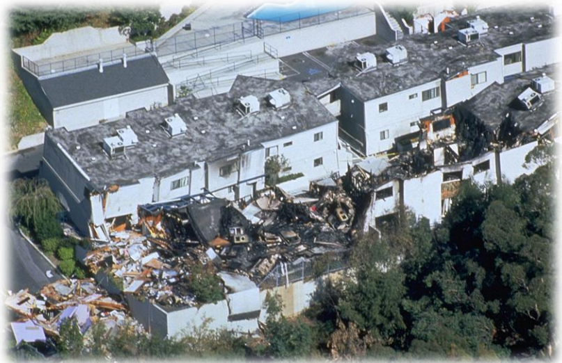
Caption: Soft Story Building Collapse at Northridge, California.
