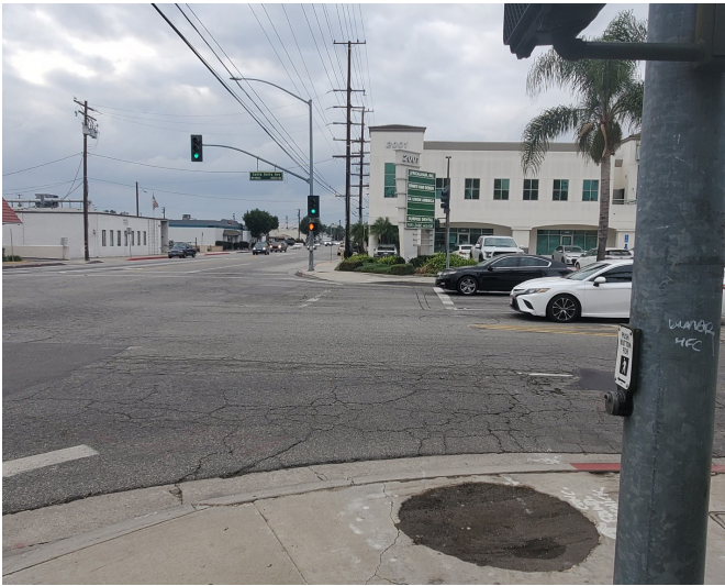
North leg crosswalk at the intersection of Santa Anita Avenue & Rush Street
