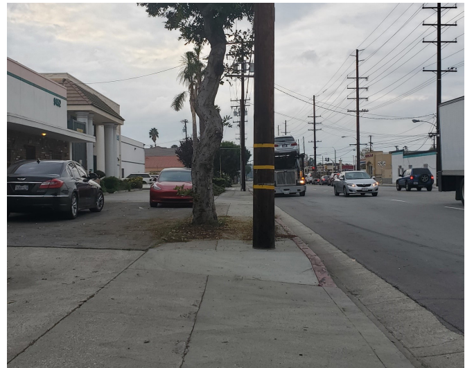
South side sidewalk along Rush Street, east of Rosemead Boulevard
