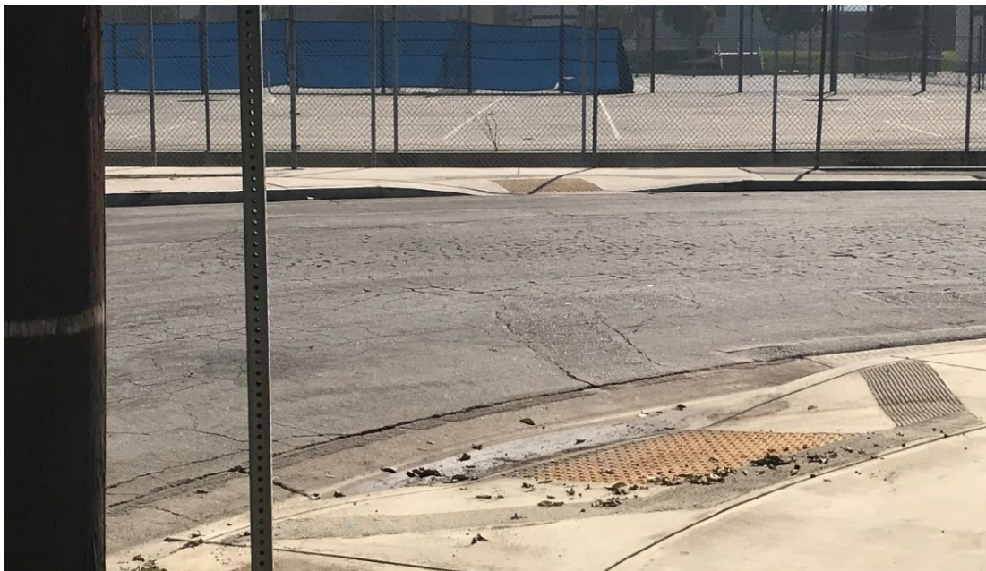
Figure 2. Pedestrian Infrastructure on Farmer Avenue
