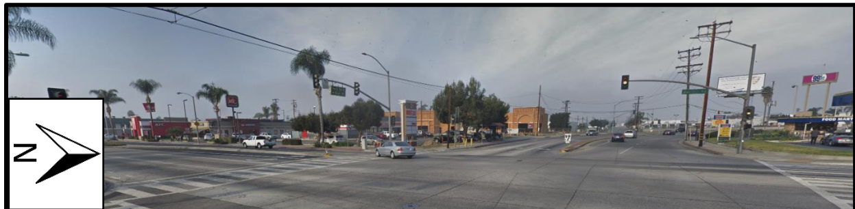
Photo of Existing Conditions for Intersection 8: Street View on Durfee Ave (WB) View at Rush St. Countermeasures S2 and S19 will be applied to this intersection.
