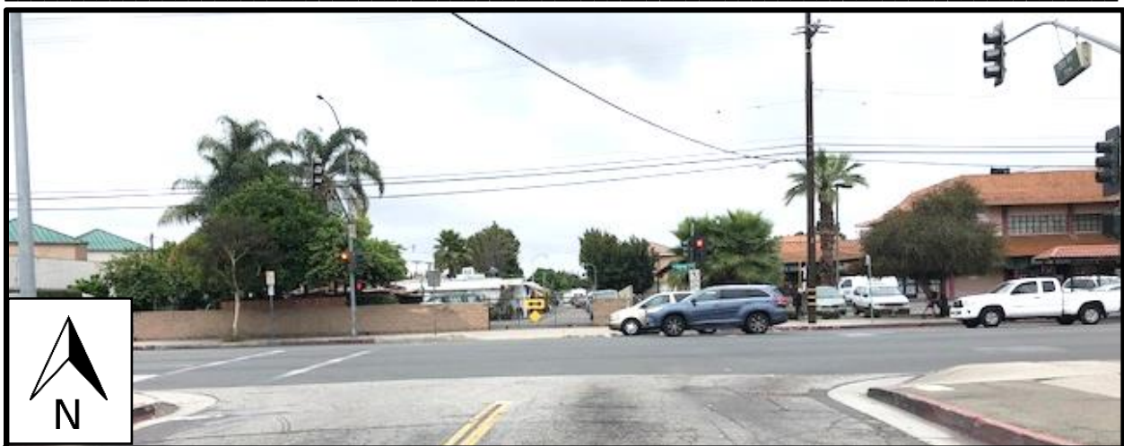
Photo of Existing Conditions for Intersection 1: Street View on Garvey Ave (WB) View at Chico Ave. Countermeasures S2 and S19 will be applied to this intersection.
