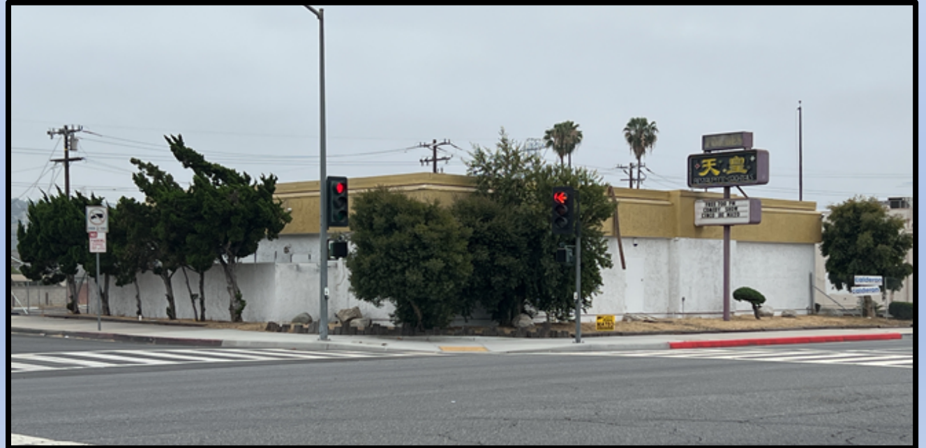
1536 Peck Road - cleaned by new owner
