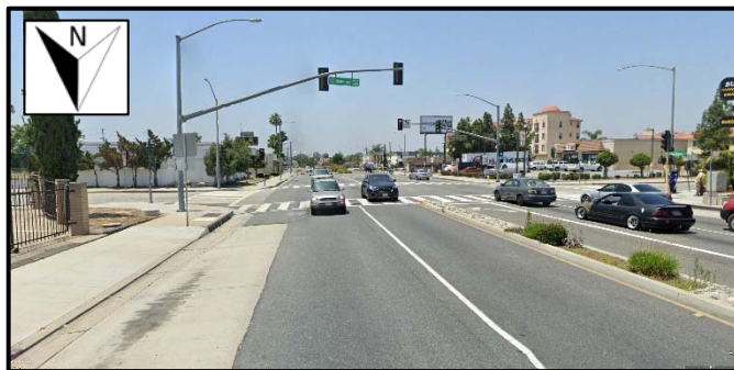
Southbound View on Durfee Avenue toward intersection.
